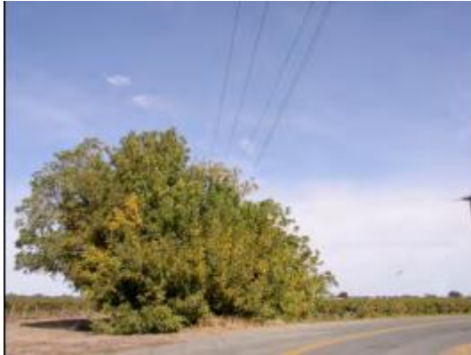
Exhibit 2-4. Conductors in vegetation reduce visibility
