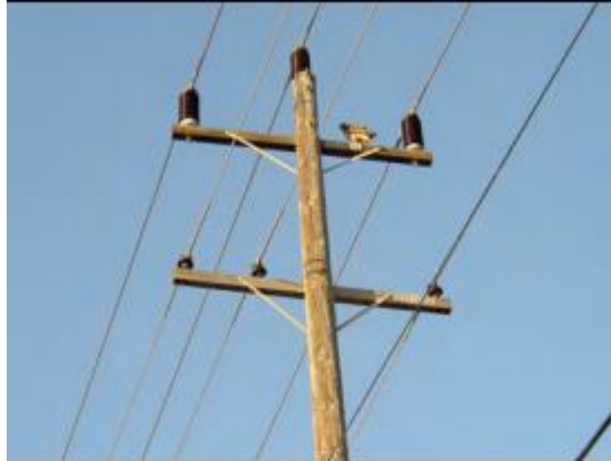
Exhibit 4-11. Double crossarm, three phase each; upper with center, lower with two on one
