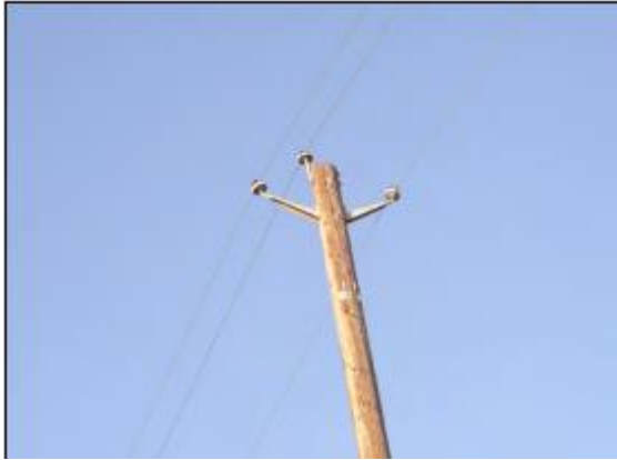
Exhibit 4-10. Three phase, one center, fiberglass crossarms
