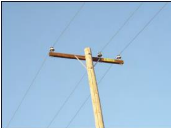
Exhibit 4-8. Three phase, two on one side
